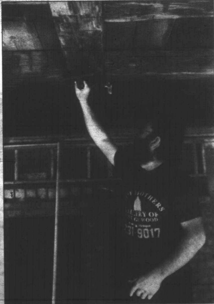
Stephen Toth uses tung oil to give a sheen to the barnwood beams in the kitchen of the home, being built by Richard Adams Russell Inc. of Ann Arbor.
